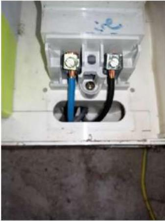
Photo Section non conforme (agcp, non accessible directement du logement)
